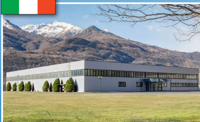
AUTOBLOK manufacturing plant Caprie-Torino
